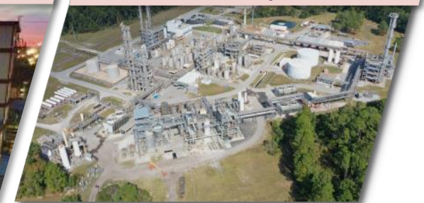
Colonel's Island chemical production site rebuild & operational
